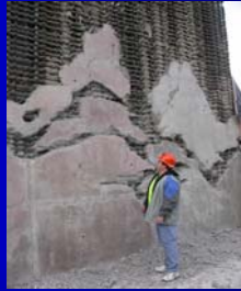
Voids in Drilled Shafts
