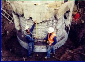
Voids in Drilled Shafts
