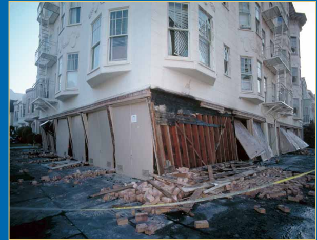
Apt. Bldg.- Loma Prieta - 1989
