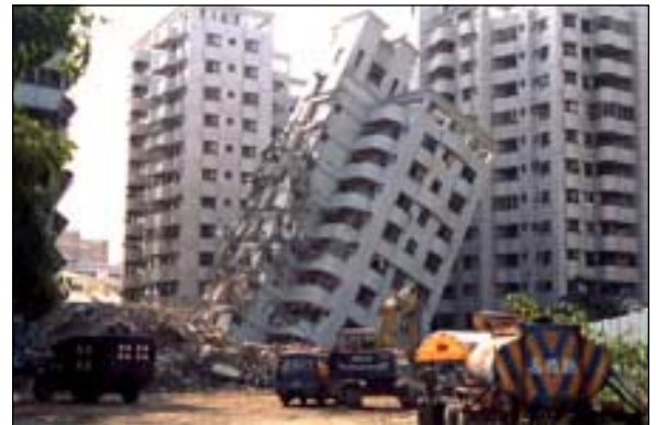
■ Figure 2. Newly constructed buildings suffered severe damage
