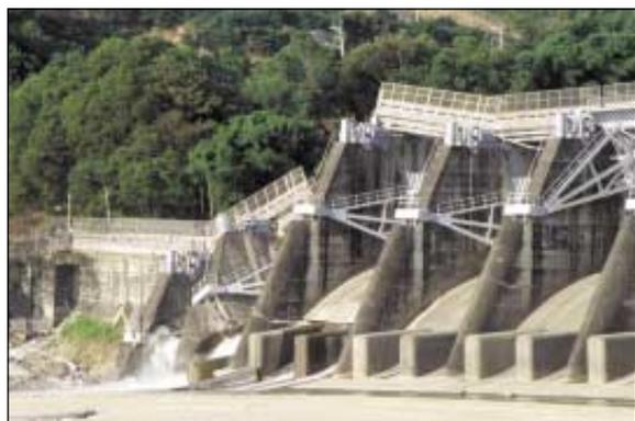
■ *Figure 1. Surface faulting caused major damage to Shih-kang Dam*
