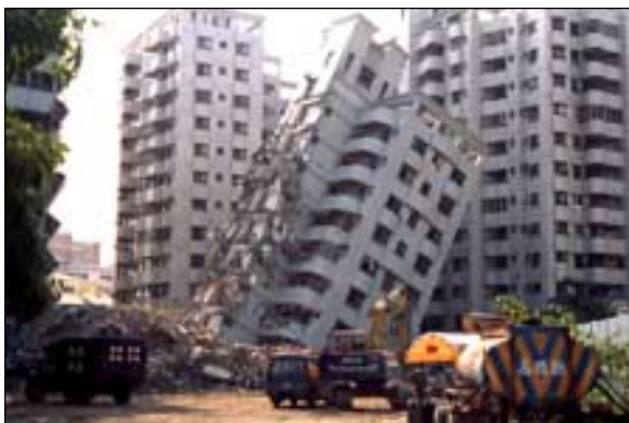
■ Figure 2. Newly constructed buildings suffered severe damage
