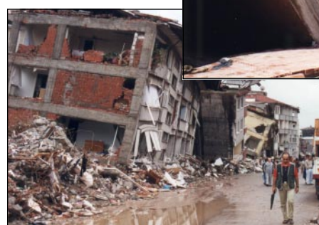
Much of the damage to reinforced concrete buildings was not surprising, nor unexpected. Engineered structures that had been built according to modern codes survived, while many non-engineered structures collapsed, causing large scale loss of life.
