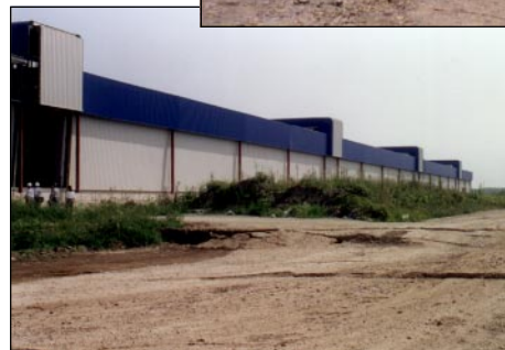
Surface faulting was common near Golcuk (above); the fault rupture is visible next to this damaged manufacturing facility, under construction at the time of the earthquake.
