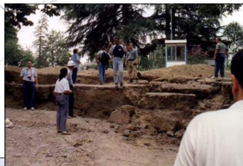
Surface faulting was common near Golcuk (above); the fault rupture is visible next to this damaged manufacturing facility, under construction at the time of the earthquake.
