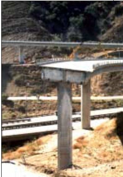
■ Figure 3. Research in spatial variation of ground motion included case studies of the SR14/I-5 interchange and other bridges damaged during the Northridge, California earthquake. Further research is needed to define the importance of these effects and to develop simplified design procedures for a broad range of bridge configurations.
