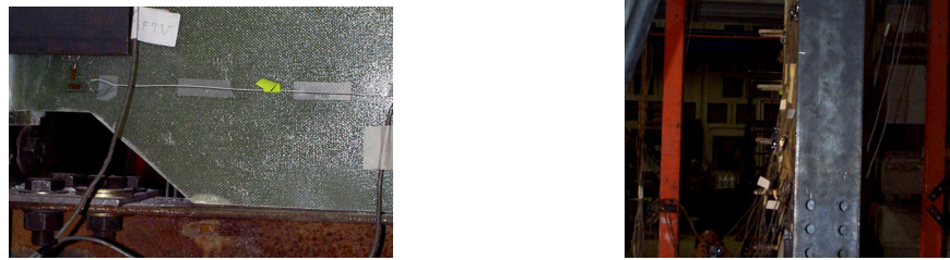
(a) Corner Crushing Damage
