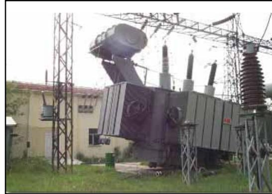
■ **Figure 1.** Transformer Failure During the August 17, 1999, Izmit, Turkey Earthquake (EERI, Oct. 99)
