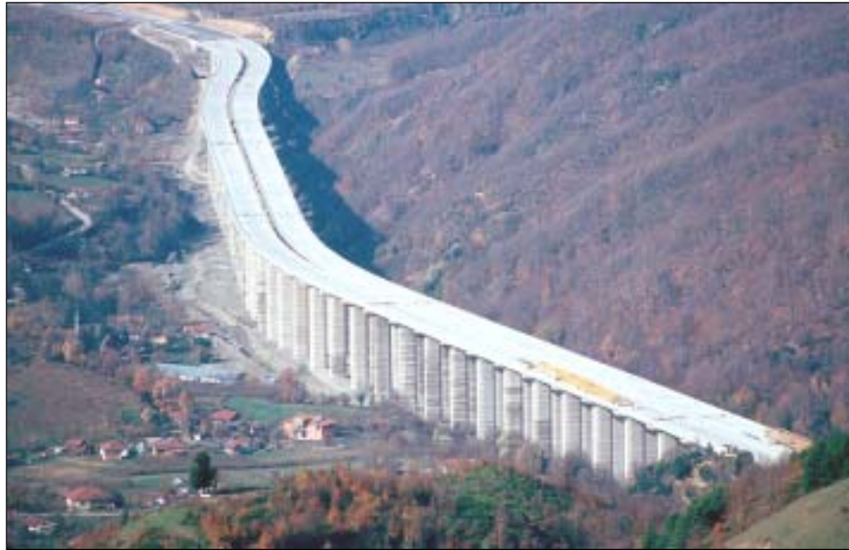
Figure 1. General View of Bolu Viaduct
