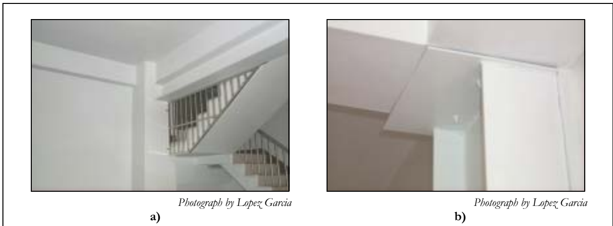
Figure 3. Non-engineered retrofit of residential buildings: (a) RC beam strengthened by a steel beam; (b) eccentric RC beam-column joint supported by a steel column
