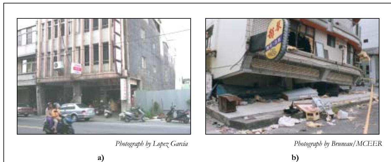
Figure 1. Typical residential building in Taiwan: (a) pedestrian corridor and open front; (b) soft story damage
