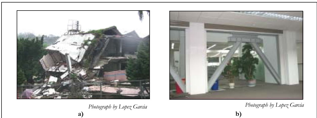
Figure 4. (a) Collapse of school building; (b) Library building retrofitted with metallic dampers
