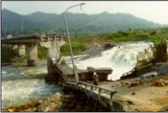
Figure 6. Bei-Feng bridge: (a) collapse of end spans; (b) after reconstruction
