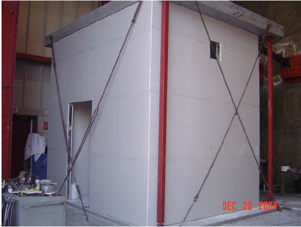
Seismic Fragility Testing of Gypsum Light Gage Metal Stud Partition Walls at PEER
