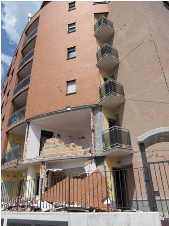
Fig. 2 Failure of the exterior wall at the second floor (left) and cracking of the exterior wall finish in the west side of the building (right)
