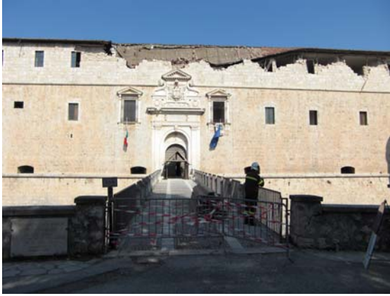
Fig. 3 Front view of the Fortezza Spagnola after the earthquake; central part (left) and right part (right). The upper part of the wall has failed at several locations. More severe damage is observed at the centre, above the main entrance, where the upper end of the wall, supporting the roof, has collapsed. As a result, the roof has sustained significant damage as well
