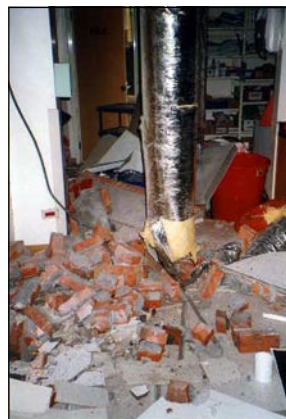
Figure 5. Interior damage in the Shiu-Tuan Hospital. Shown are (top) fallen brick inside the hospital and (right) a damaged interior glass brick wall.
